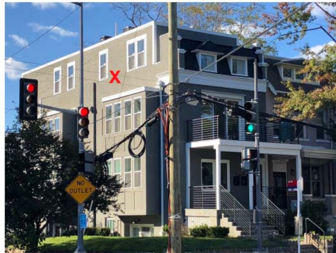
October, 2018 Site Visit
